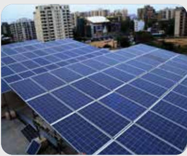
35kW p Installation, Gurugram Industry/Sector : Corporate Office
