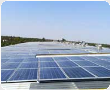
330kW p Installation, Jaipur Industry/Sector : Stone
