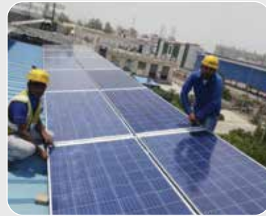
55kW p Installation, Kundli Industry/Sector : Engineering
